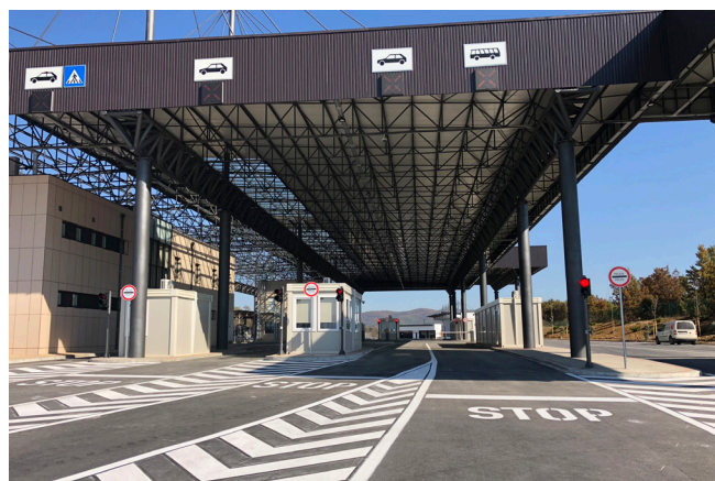
2018. UNOPS Kosovo In the picture, the crossing point of Merdare.
